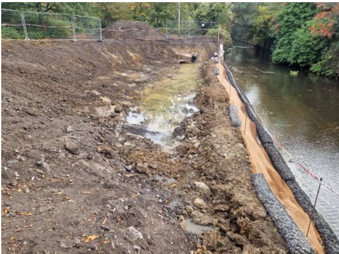
Partially completed excavation as part of the Mereway river restoration project
